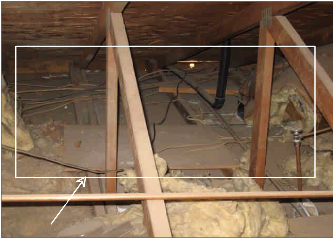
Figure Set 46 - There is a lack of insulation in a living space
