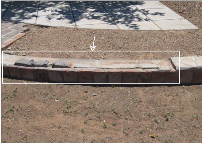
Figure Set 7 - The walkways or decorative edging are damaged in various areas and should be repaired or replaced
