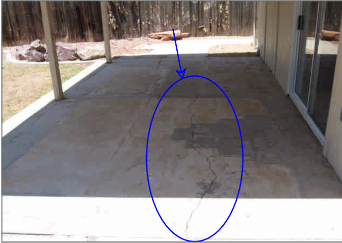
Figure Set 11 - The patio concrete is cracked but appears to have settled and is not cracking further
