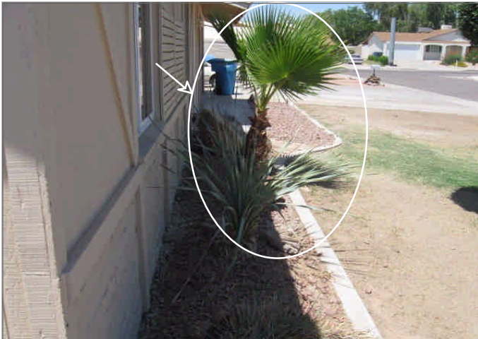
Figure Set 2 - A tree or bush that is adjacent to the foundation should be monitored
