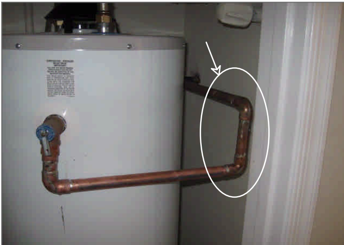
Figure Set 24 - The discharge pipe from the relief valve has been incorrectly plumbed uphill
