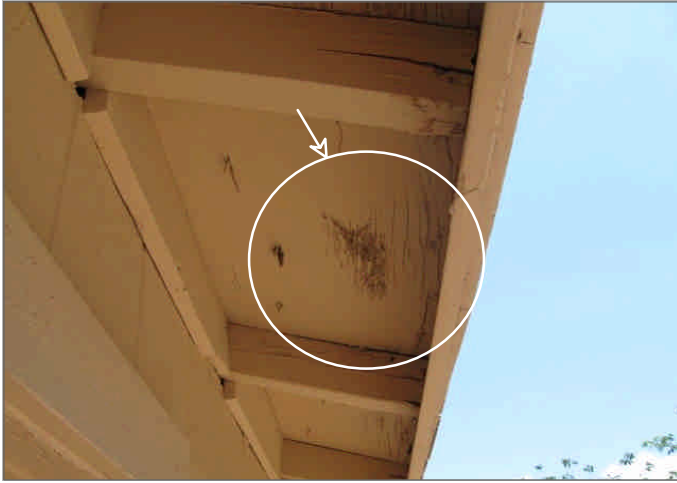
Figure Set 6 - Sections of the eaves and soffits are weathered and should be serviced
