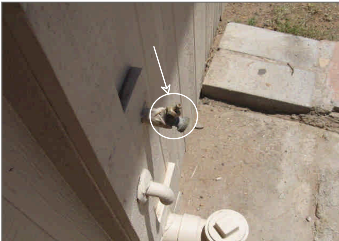
Figure Set 19 - A hose bib is missing a handle which should be replaced
