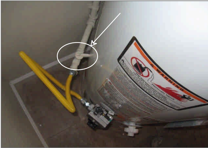
Figure Set 23 - The shut-off valve for the gas water heater would be difficult to access
