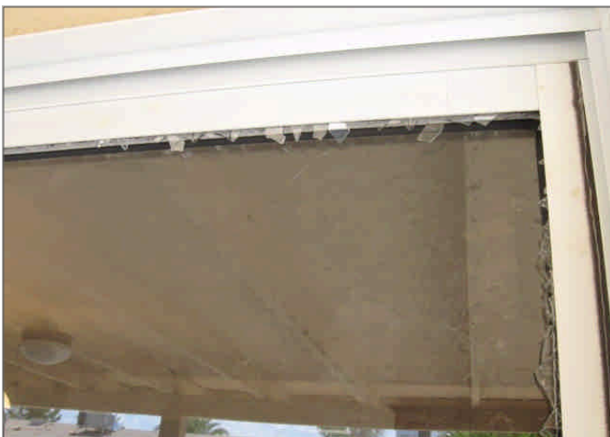
Figure Set 10 - One of the glass panels in the slider is broken
