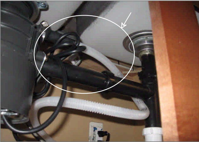
Figure Set 43 - The dishwasher does not have a high loop on the drain line
