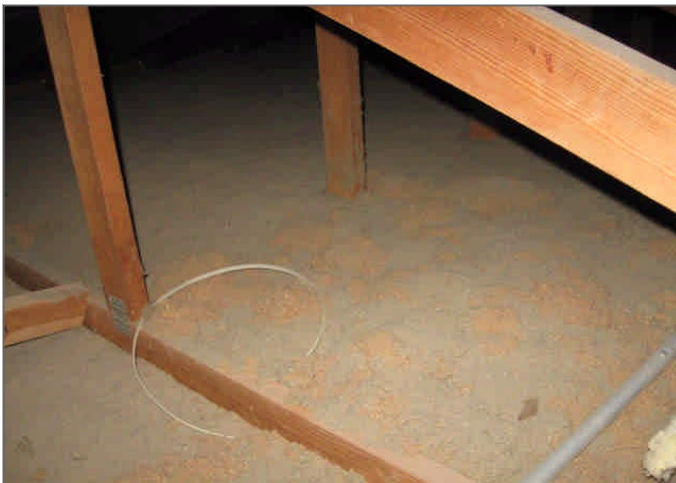
Figure Set 47 - The attic is insulated with approximately three-five inches of blown-in cellulose
