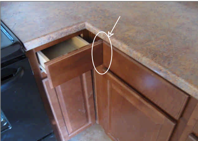
Figure Set 42 - A cabinet door does not open completely because it hits the adjacent drawer
