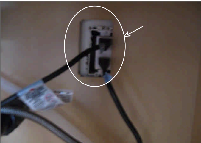
Figure Set 39 - There are electrical outlets that are missing outlets covers and present a safety risk
