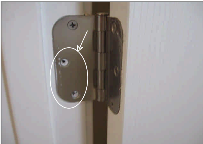
Figure Set 32 - One or more doors are missing screws in the hinges that should be installed
