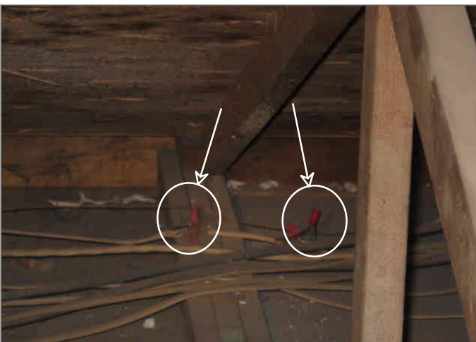
Figure Set 45 - An electrical connection has been made incorrectly outside of a junction box
