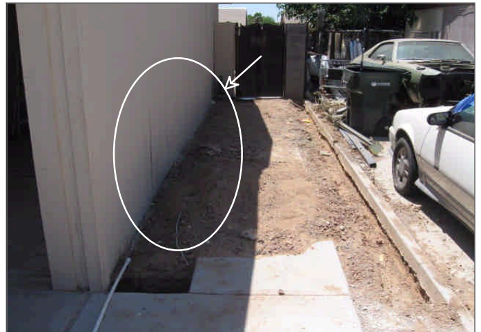
Figure Set 4 - The siding on portions of the house is in direct contact with or too close to the ground
