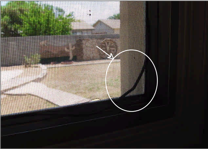
Figure Set 38 - A window screen in the master bathroom is torn and should be repaired
