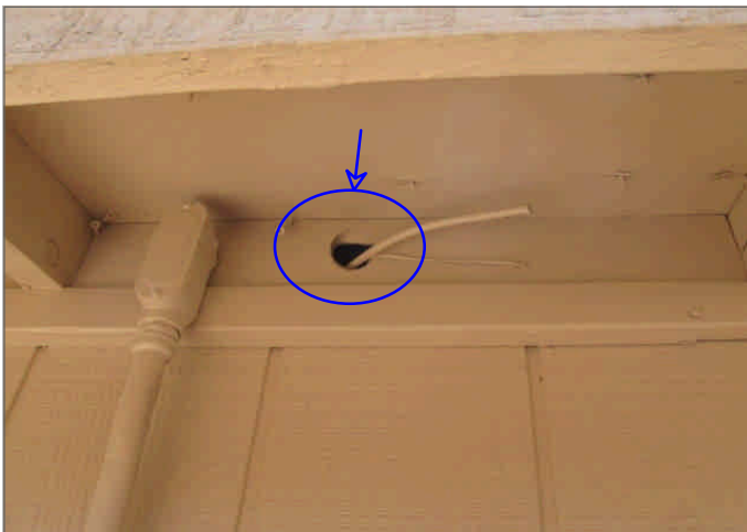
Figure Set 5 - There are cables run through a bird screen that should be sealed to prevent bird or pest entry
