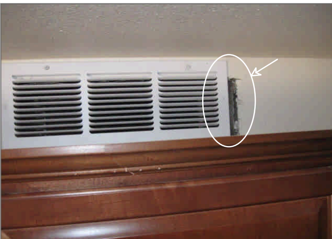
Figure Set 30 - A wall register is not trimmed correctly as indicated within the report and should be repaired
