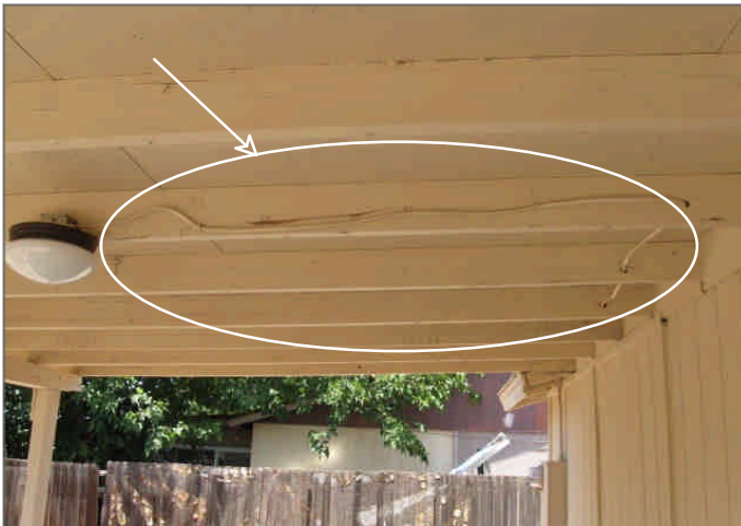
Figure Set 12 - There are electric lines on the exterior that are not in conduit and could become a safety hazard
