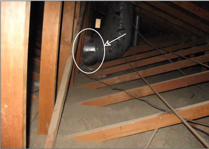
Figure Set 28 - Insulation or vapor retarders in unfinished spaces were observed to be missing and require servicing
