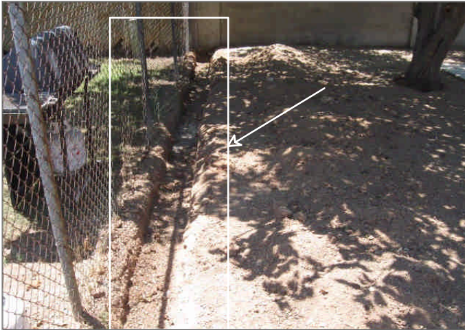
Figure Set 8 - There are open trenches for block walls that present a safety issue for tripping until the block is laid
