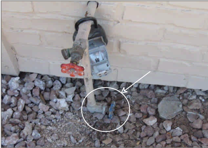
Figure Set 18 - The main water shut off valve leaks and does not fully close and should be replaced
