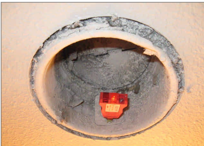
Figure Set 35 - The main bath exhaust fan was not installed and could not be tested
