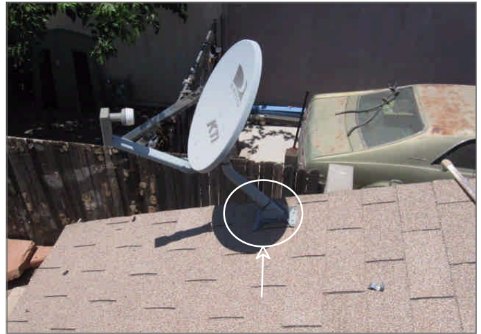
Figure Set 16 - There are roof penetrations that should be sealed with mastic to prevent moisture entry
