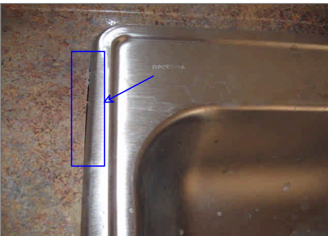
Figure Set 40 - An open seam between the sink and the counter top should be caulked
