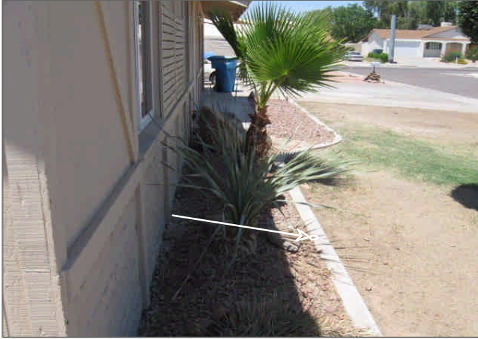
Figure Set 1 - Minor adjustments of the surface grading to direct surface moisture would be beneficial
