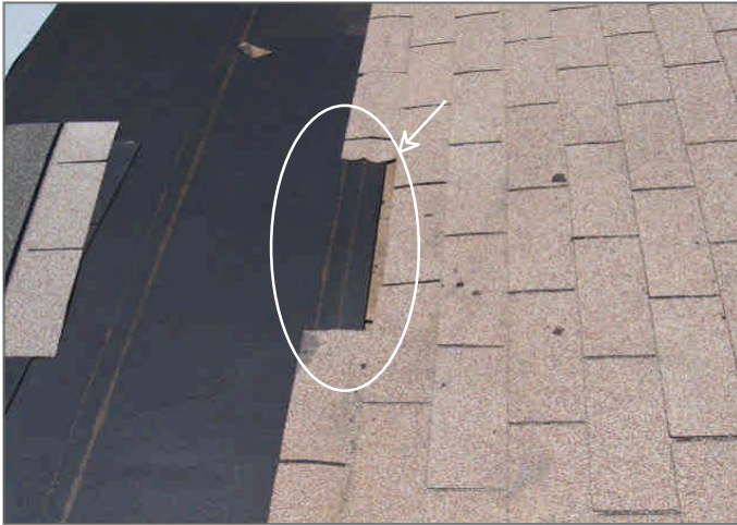
Figure Set 13 - Some shingles are loose or missing and should be repaired or replaced
